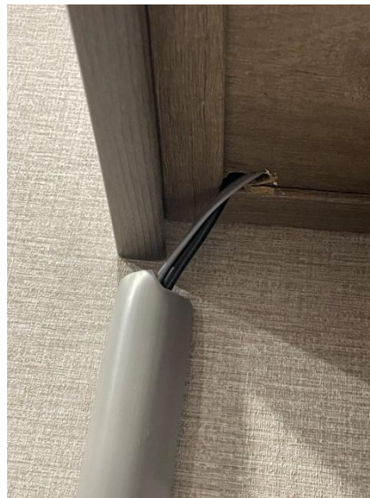
Oblong hole drilled under cabinet for cords
