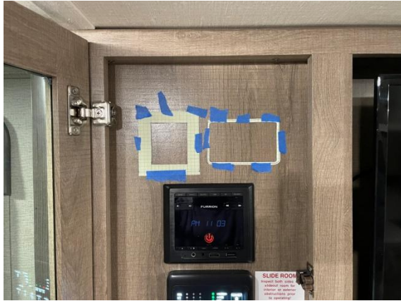
Stencils in place
