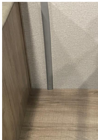
Bench cover is cut to fit around wiremold
