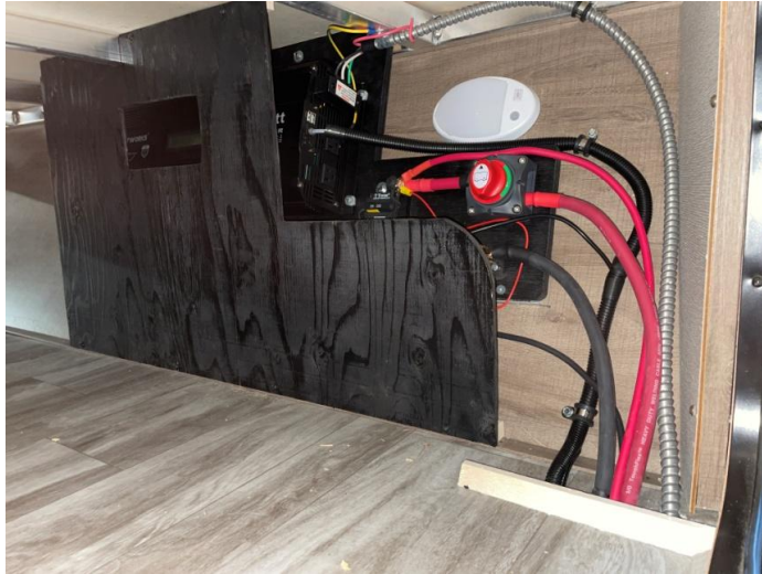
Inverter panel in place. Note 7\frac{3}{4} " 1x1 mount in place for cable panel
