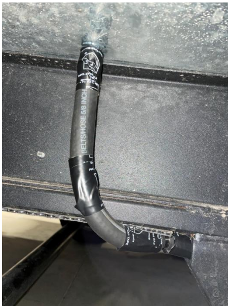
More heater hose as protective sheath
