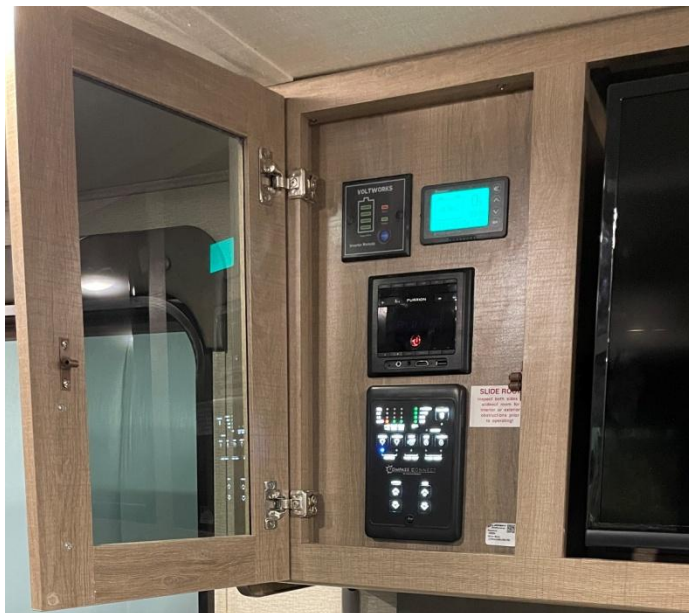
Panel and monitor in place and tested
