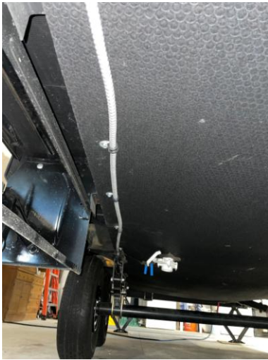
MC cable mounted with clamps
