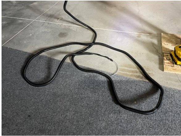
Both cords inserted into split loom and closed up
