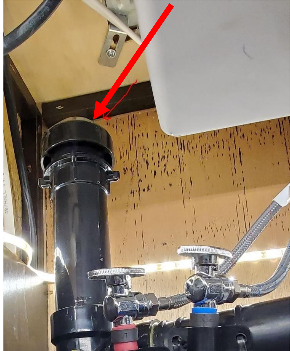
Air Admittance Valve (AAV)
